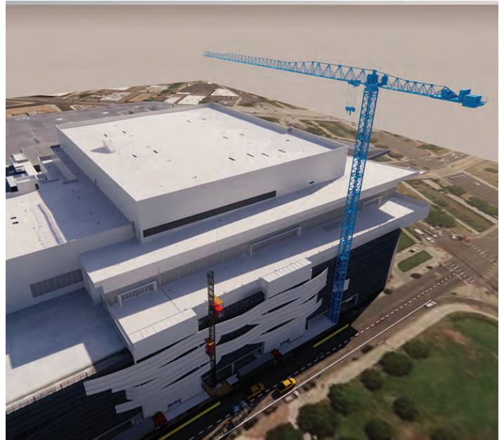
ALL IMAGES: The 3D model of Comansa 37.5-t 21LC750 tower crane for a jobsite at the Colorado Convention Centre in Denver, USA.
