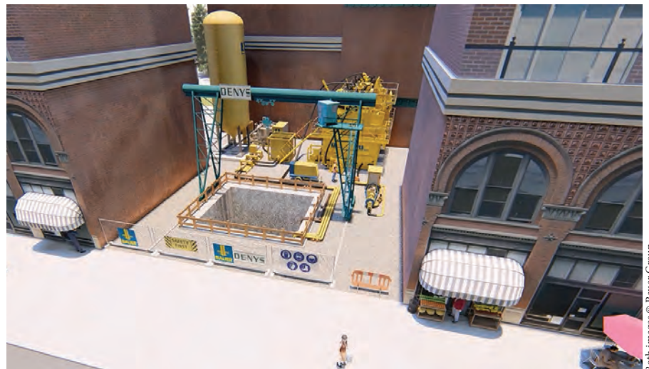
With Bauer Cube System, the surface impact of cutting sites can be reduced to a minimum. This is because the minimally invasive system only requires a comparatively small access point to an existing microtunnel or auxiliary tunnel. The actual work is carried out underground, essentially invisibly.
