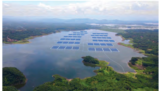
When completed, the Cirata Floating Photovoltaic Power Plant will provide enough electricity to power 50,000 homes and offset 214,000 t of carbon dioxide emissions per year.
